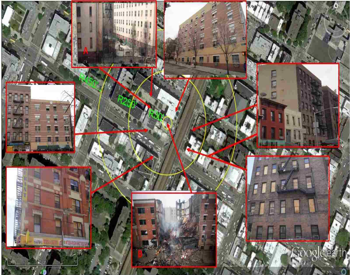
Figure 41 Associated damage between 30 to 250 ft [9]
