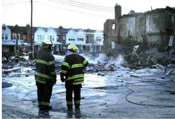
Figure 33 The demolished houses in Allentown's accident [6].
